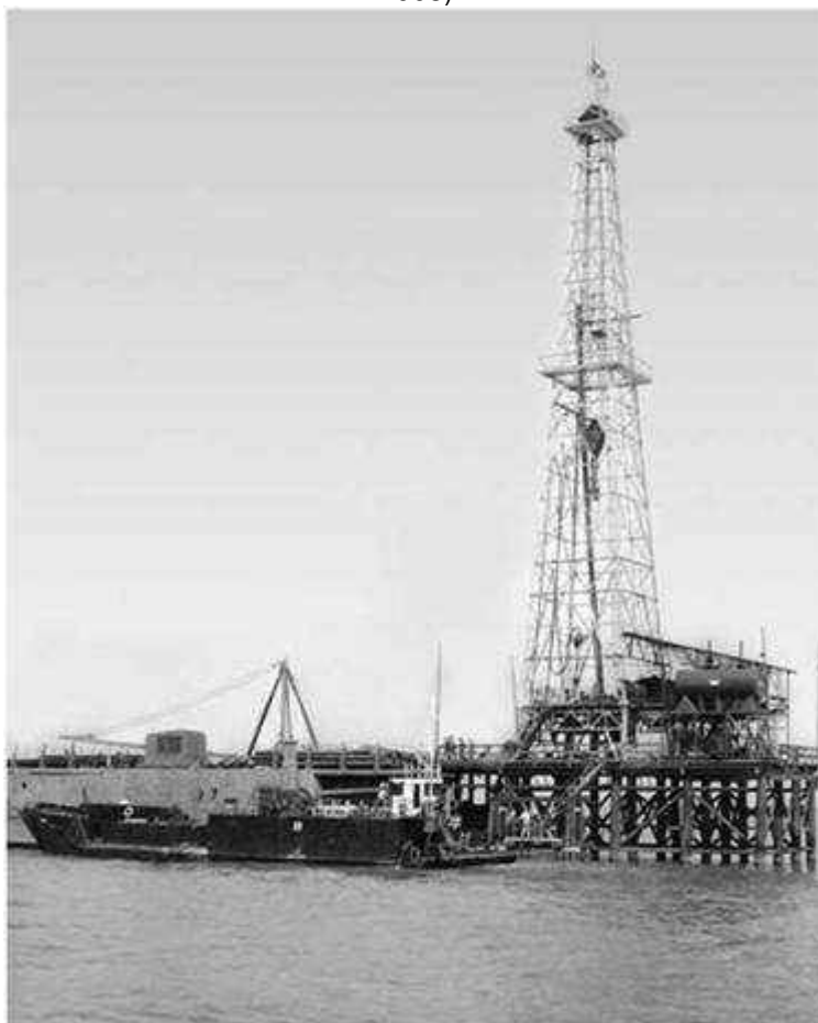
Figura 2.3 – Primeiro poço “out of sight of land” – Kerr Mcgee Rig 16 (extraída de Smith, 2008)
