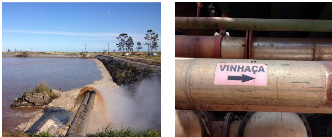
(a) (b) Figura 3.12 – Coleta de vinhoto na Usina Canabrava (a) e Coagro (b).
